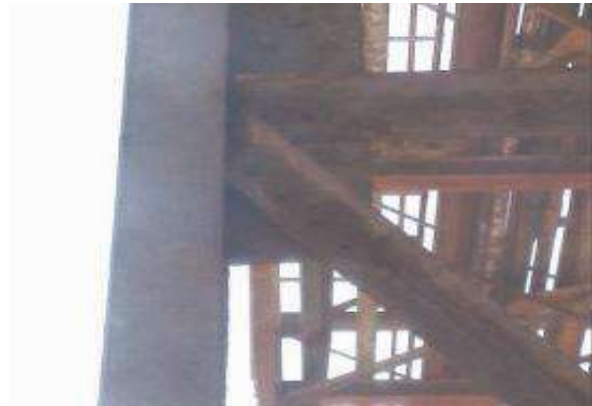
Figure 7 Deformation of bracing system and buckling column.
