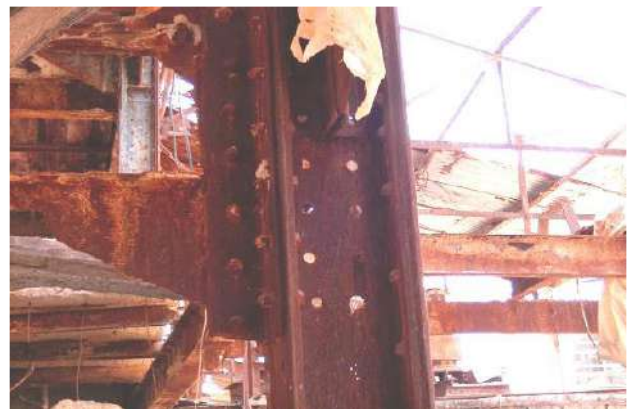
Figure 4 Damage in the assembly system.
