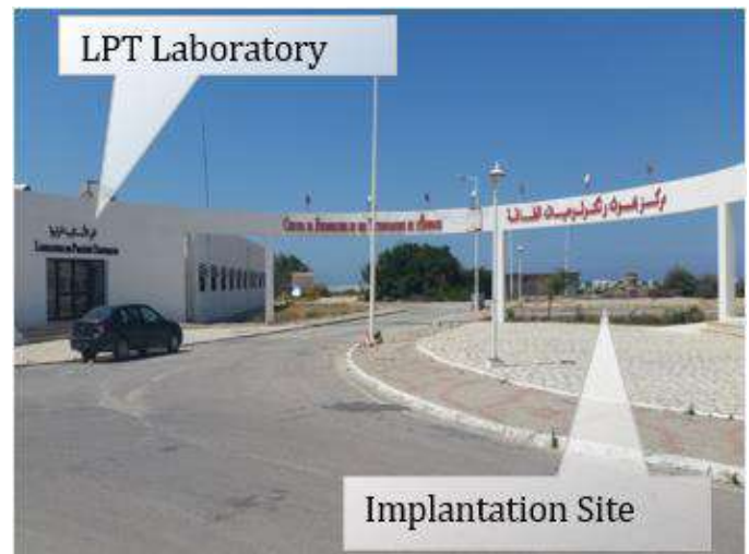
Figure 1. Laboratory Site and the platform of our installation.
