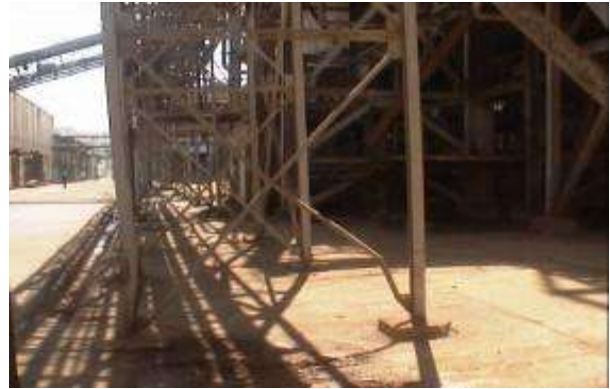
Figure 7 Deformation of bracing system and buckling column.
