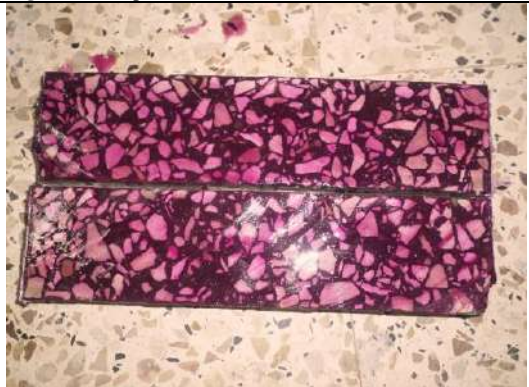
Figure 5 : detection of the carbonated zone
